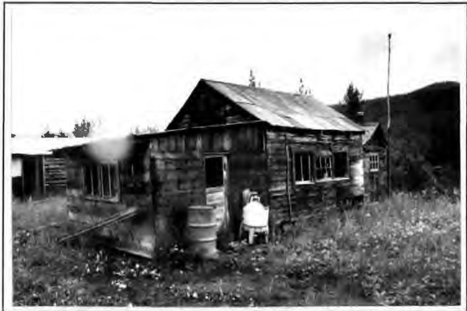
Figure 119. The Stuver Shop/Shawn Flemings House, 1993. The view is looking northwest.
